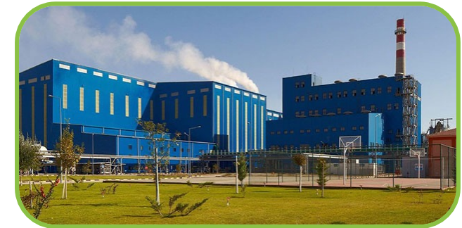
Eti Soda : ~ 1 million mtpa expansion
